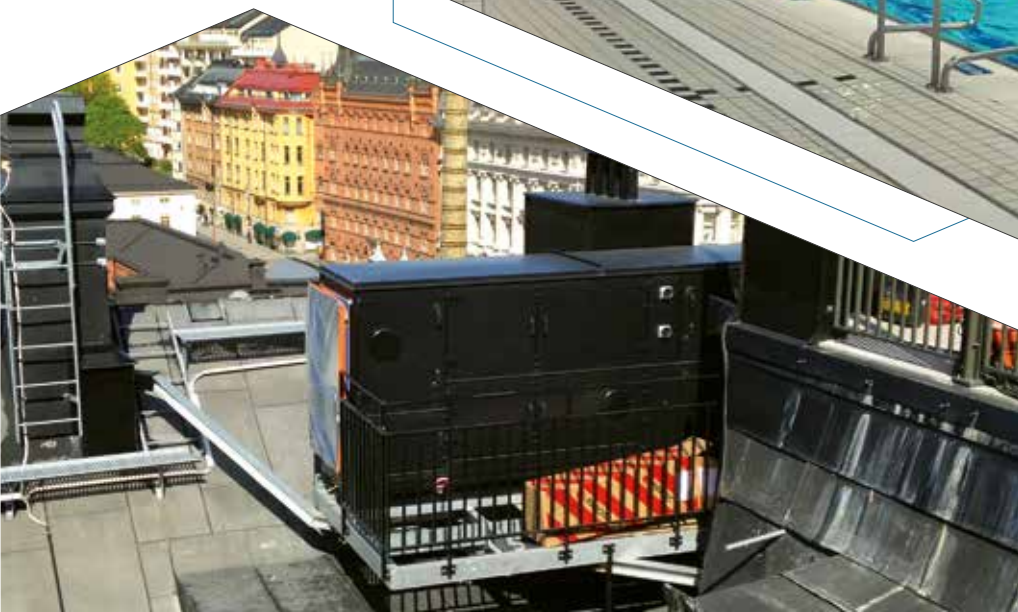
Pool Line rooftop unit with control cabinet, Strandvägen, Stockholm.
